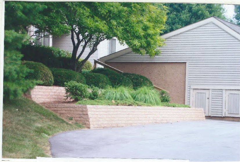
Railroad Ties replaced with E.P.Henry Brick 2005 & 2006
