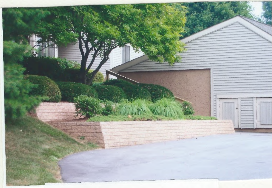
Railroad Ties replaced with E.P.Henry Brick 2005 & 2006
