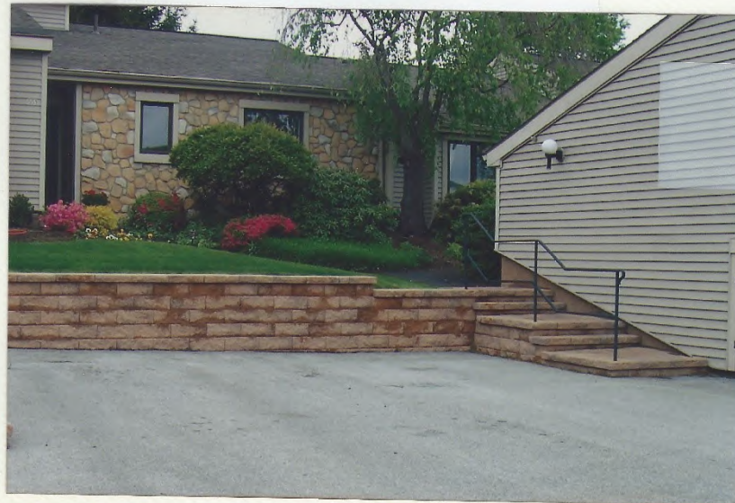
Railroad Ties replaced with E.P.Henry Brick 2005 & 2006
